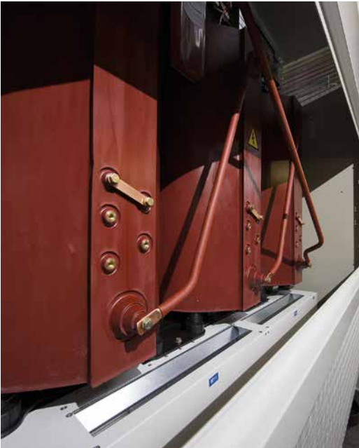
Force-ventilated transformer in IP31 enclosure
